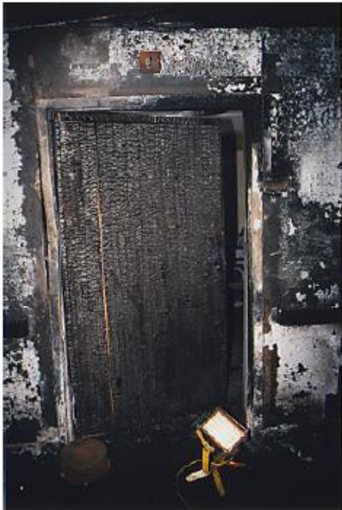
Figure 6 – Exterior of closed door of patient room. (NFPA)
